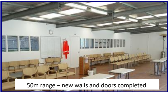
50m range during construction of new walls
