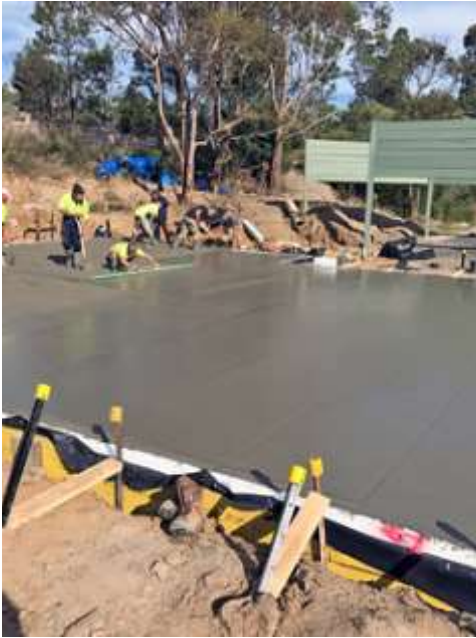
Range 2&3 new slab poured and construction begins.
