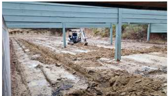
Digging trench lines in preparation for cables and concrete (March 2015)
