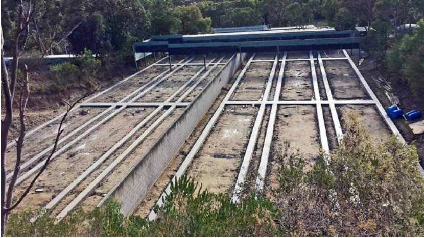
Range from top of Mounds – Concrete completed.
