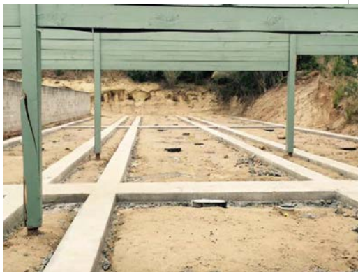
Concrete strips drying
