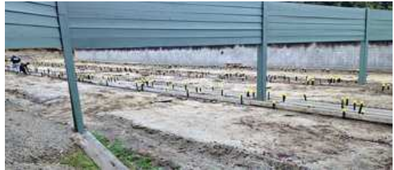
Form work commenced for the laying of air/electrics and concrete (April 2015)
