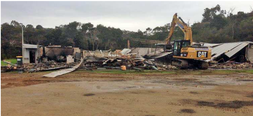
Excavator clears away the damage
