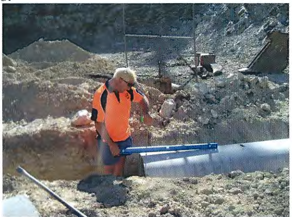
Vin Bourke setting levels for drainage
