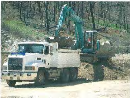
Excavation work carried out by V & L Excavations
