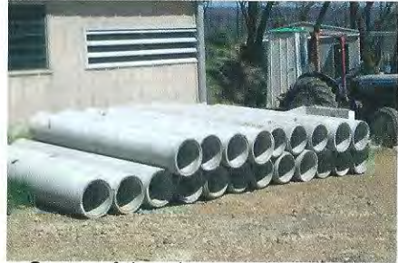
Some of the pipes and headwall supplied by Rocla
