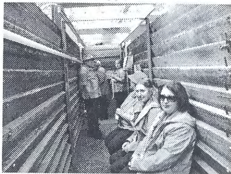
Workers in the tunnel
