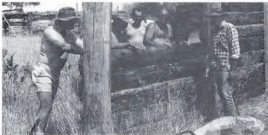
Building 25mt Range Wall
